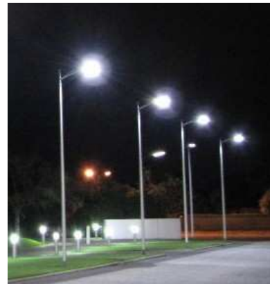
LED Street Lighting
